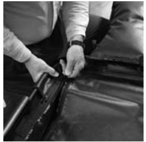
15. It is recommended that zippers be started, beginning with the right front, then progress to left front.
